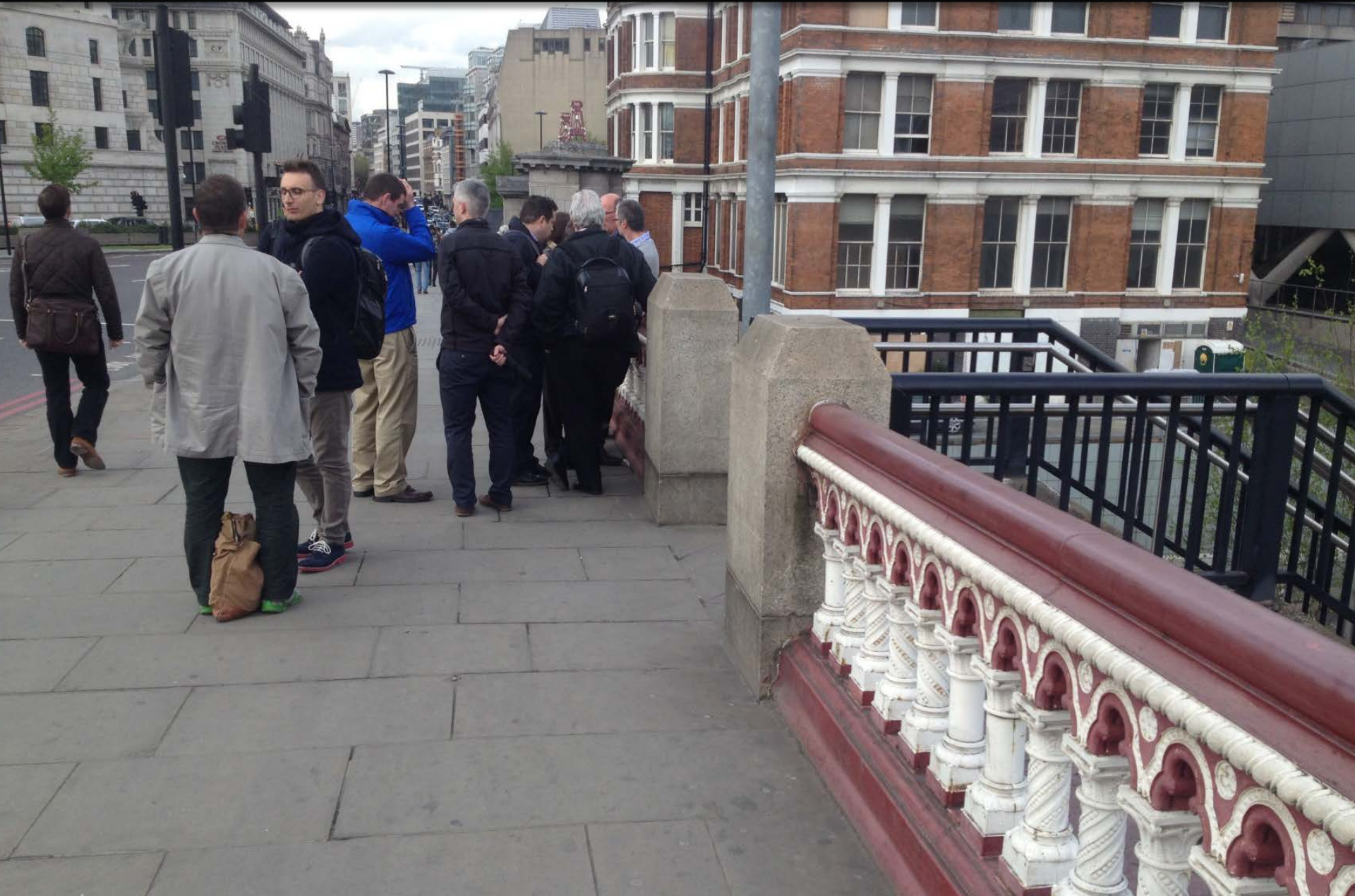
Existing entrance to stairs on Blackfriars Bridge.
