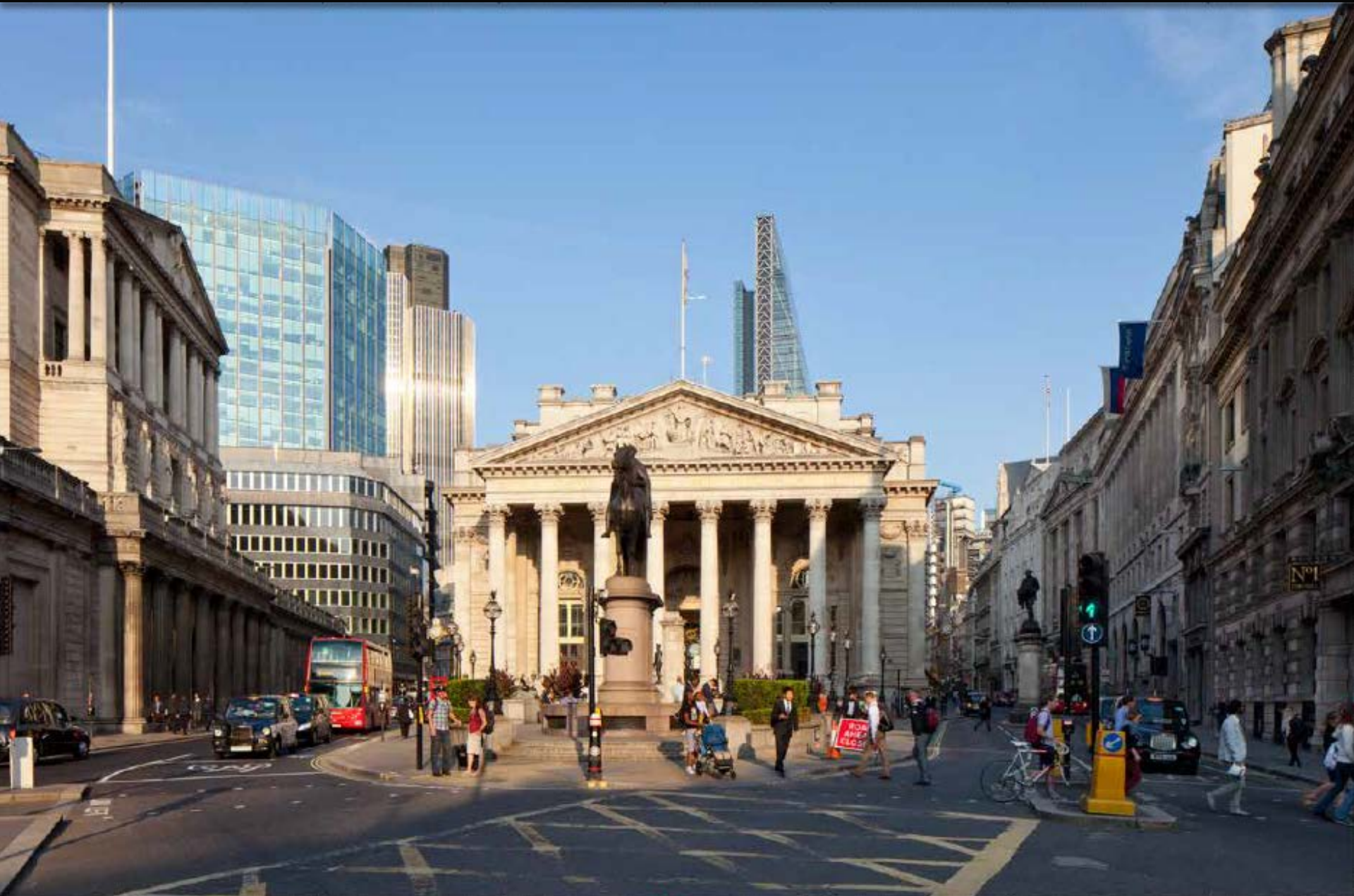
Existing view - Bank Junction
